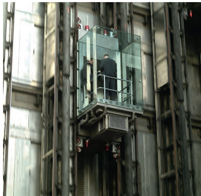
Figure 5.18 A lift needs a powerful motor to raise the car when it has a full load of people. The motor does many thousands of joules of work each second.
